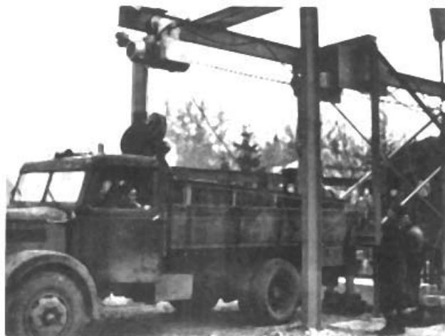
Fig. 5 Transportation of the tank of the eel-rack at Siófok.
